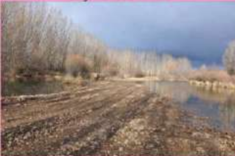
Works recently completed
